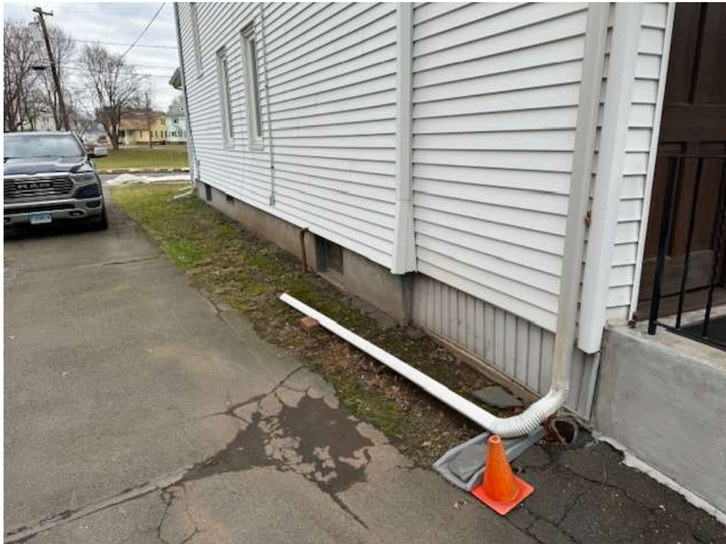
View of right foundation wall.
